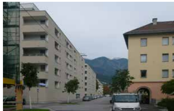
The road side of the block of flats in the Sebastian-Scheel-Straße, viewed from the southwest, shows the clear definition of road space with well-usable loggias for the inhabitants and a raised ground floor, at a distance of more than 2 m (height of the window breast) from the road. Photo: M. Schönherr
